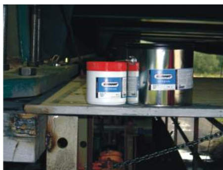
chuck plates being coated with MM 1018
