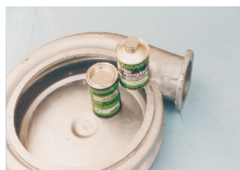
repair of blow holes on a pump housing
